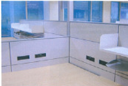
Installed Thick Tile Brackets with Outlets
